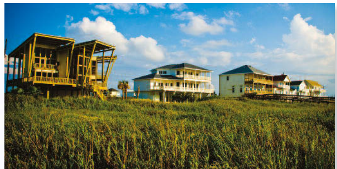
Rebuilding efforts along the once pristine Texas shoreline (above) are under way following the devastation caused by Hurricane Ike (shown below).
