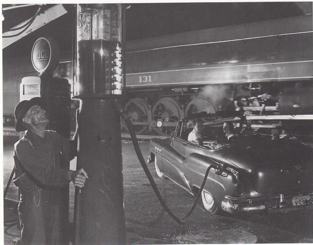
Sometimes the Electricity Fails, Vesuvius, Virginia, 1956
