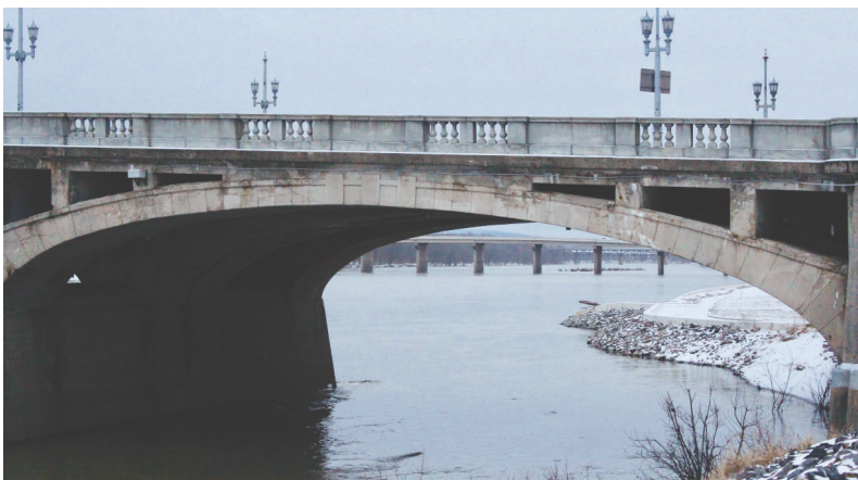
A bridge, under the bridge, over the water.
