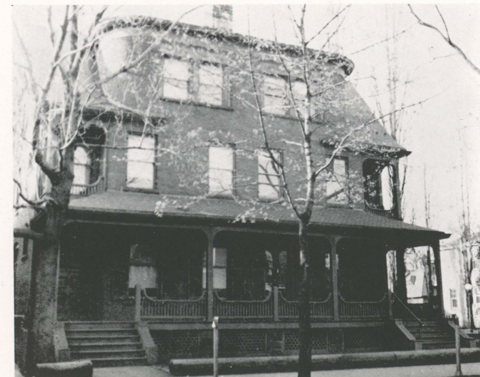
THE FORMER STODDARD HOME Recent Addition to the Campus
