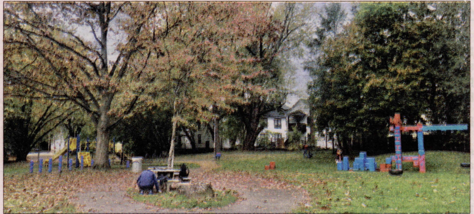
Charles Street Park, located at 26 Irving Place, pictured at the beginning of cleanup.
