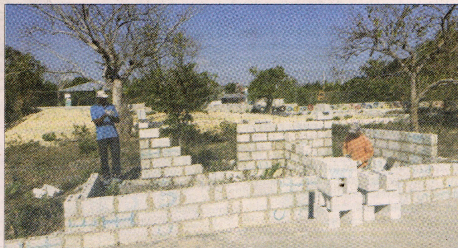
In the Dominican Republic, students assisted with the construction of buildings.
