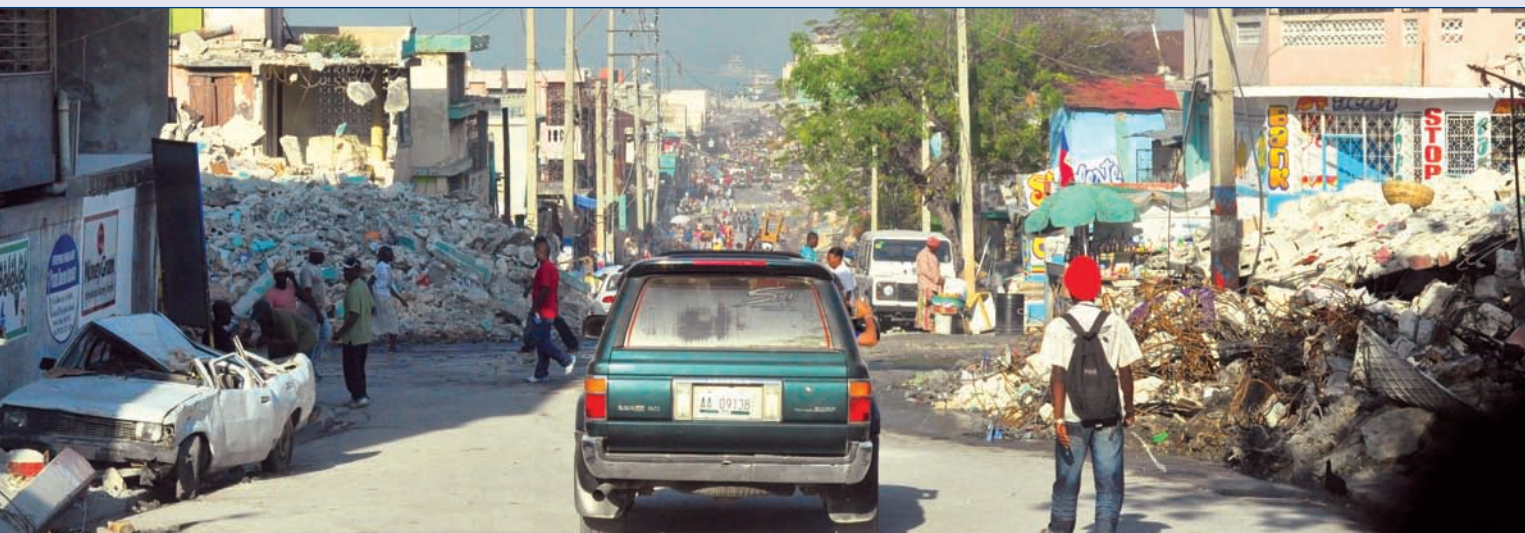
A street in Port-au-Prince, Haiti, after the earthquake. PHOTOS COURTESY OF DR. ASIF ILYAS
