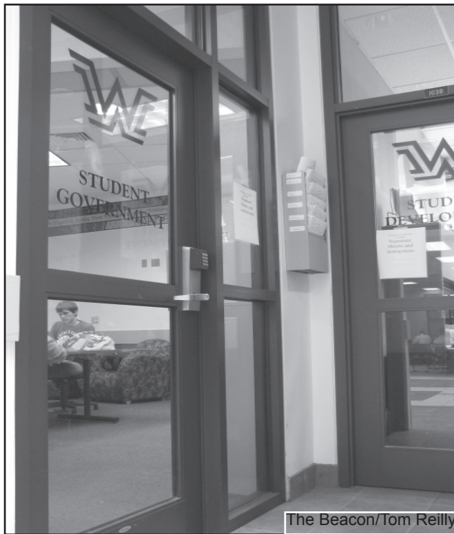
Current lock system to be replaced located outside the SG office on the first floor of the sub.
