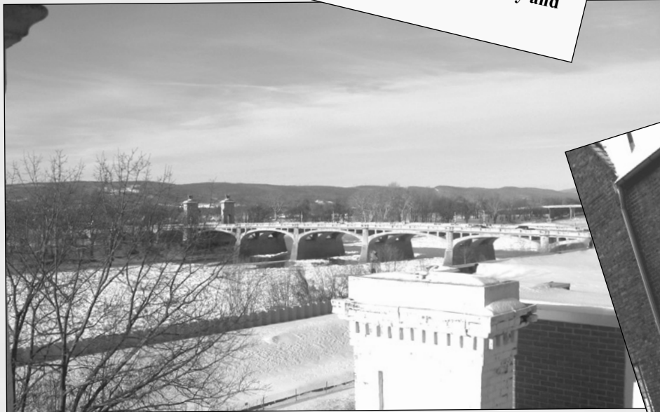
The Susquehanna River was a log jam of ice and snow after Wednesday's storm, which dumped over two feet of snow on the Wyoming Valley.
