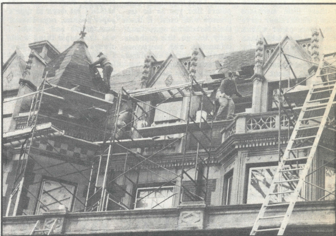
Workmen make repairs to the roof of the Conyngham Student Center.
