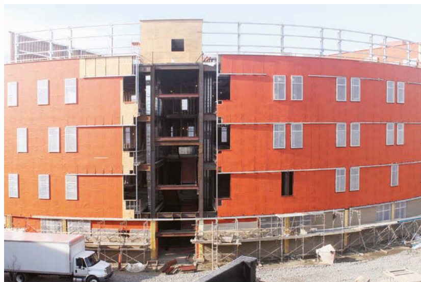
Nov. 23: Exterior walls are installed.
