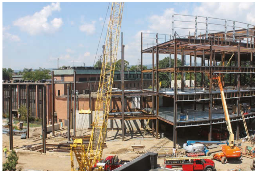
Aug. 23: Steel beams form the shape of the building.
