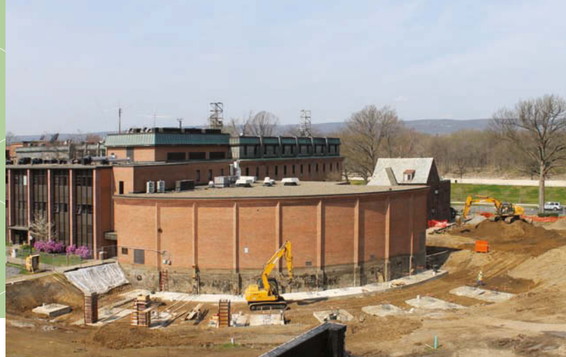
March 23: The site is prepared for construction.
