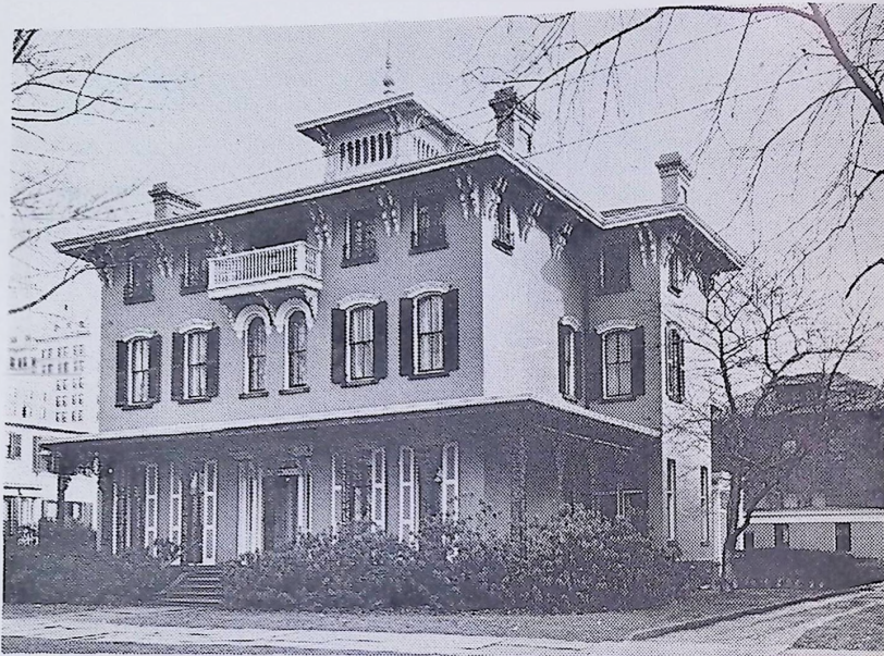
72 SOUTH RIVER STREET
