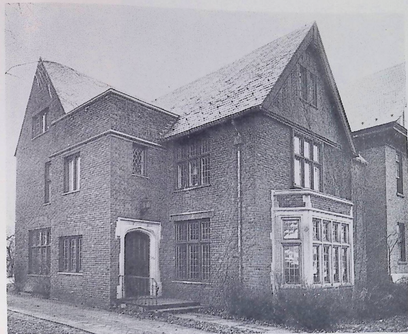
146 SOUTH RIVER STREET
