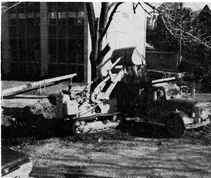
Moving mountains and mole hills with a diesel-powered traxxavator.
