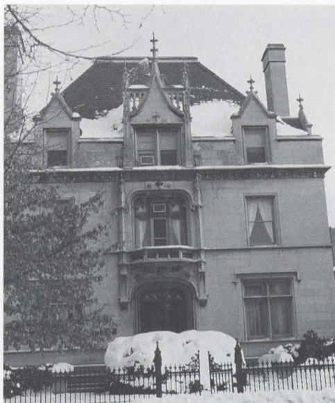
Below Left: A view from River Street shows Evans Hall and other historic buildings.
