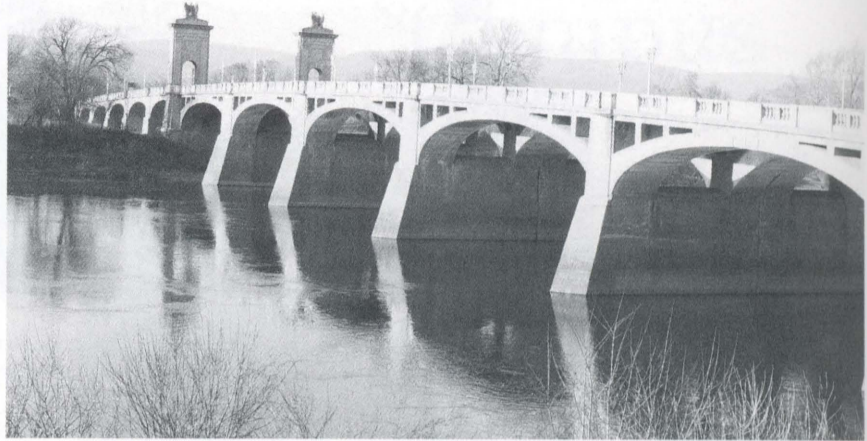
Right: The Market Street Bridge is a familiar sight to those who dorm along River Street. The impressive structure was built in the early 1930's, and has withstood two major floods.
