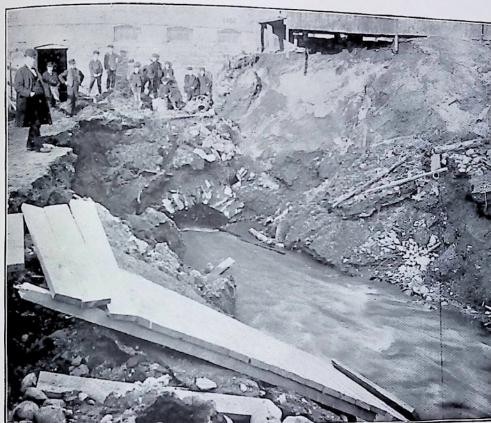
EAST PITSTON—Damage by flood on Railroad Street, showing cave-in of Stone Culvert.
