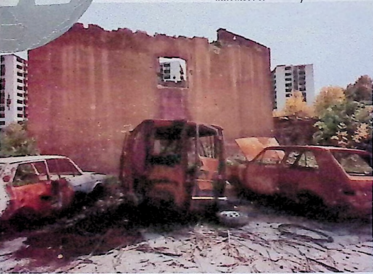
▼ Bombed-out buildings and destroyed automobiles in Sarajevo
