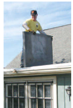
Jim Bochicchio removes debris from a roof.
