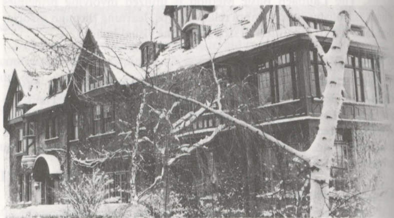
Chase Hall on South River Street houses the Admissions office.
