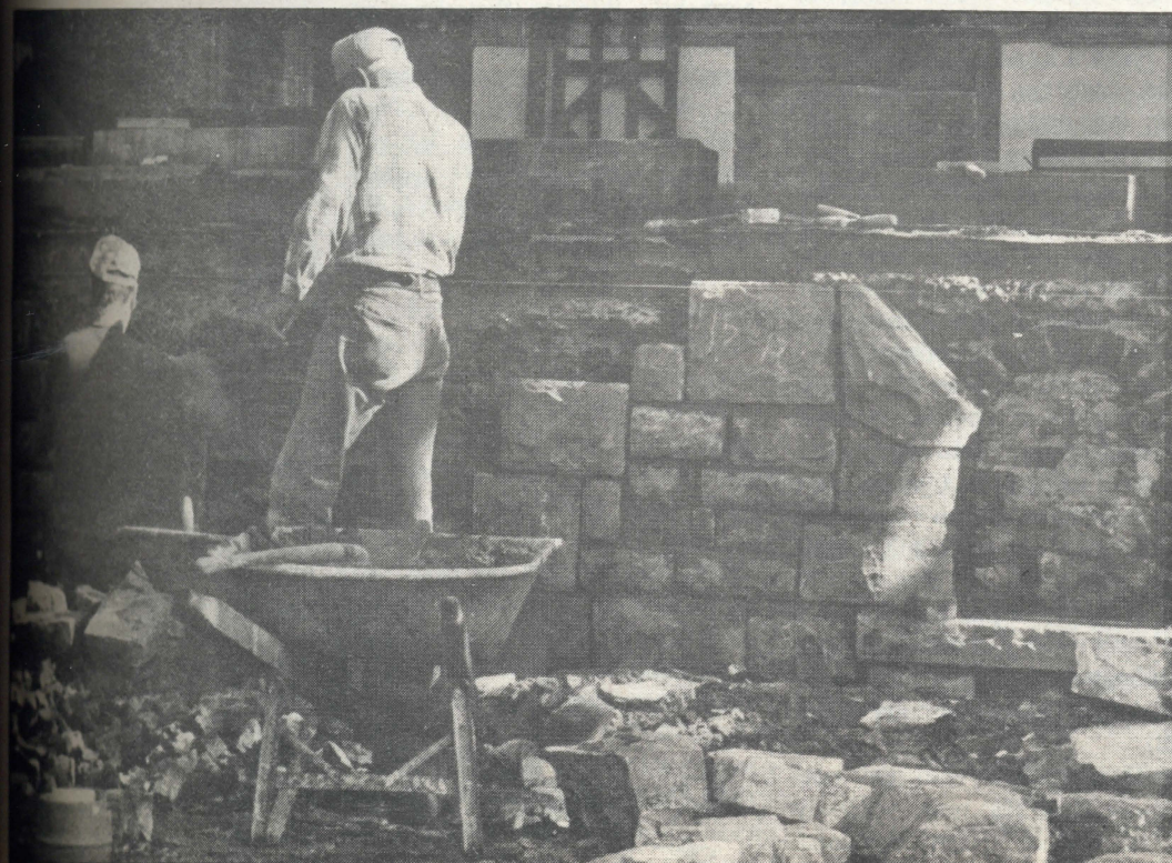
Workers rebuild the stone wall outside Chase Hall. According to John Pesta, director of Purchasing, the brick behind the stone was crumbling and the stone wall was beginning to pull away.
